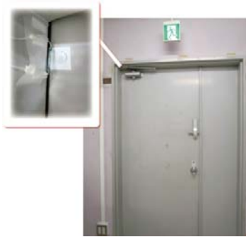
figure 6. A reed switch at the entrance door.
